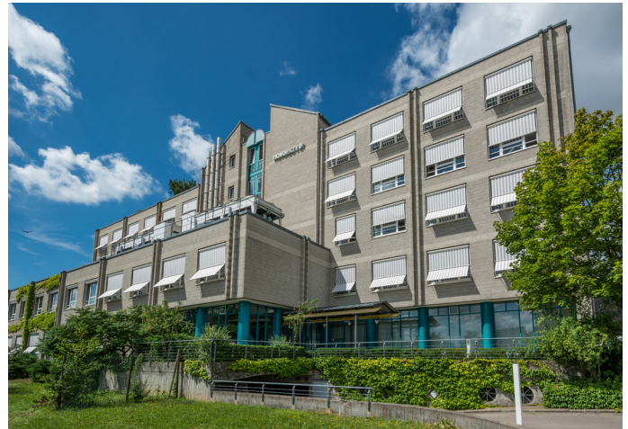
Novotechnik Ostfildern (Germany), Production
