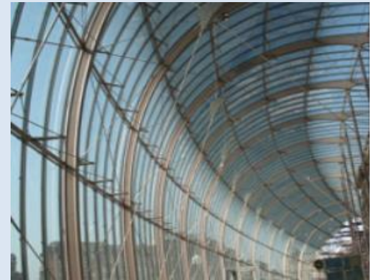
Strasbourg Railway Station facade structure 400 tons of steel structure
