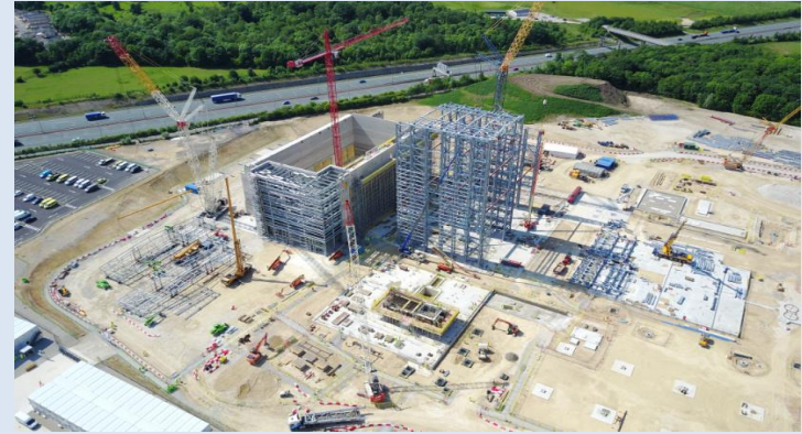
Ferrybridge Waste to Energy Plant, United Kingdom 6 500 tons of steel structure
