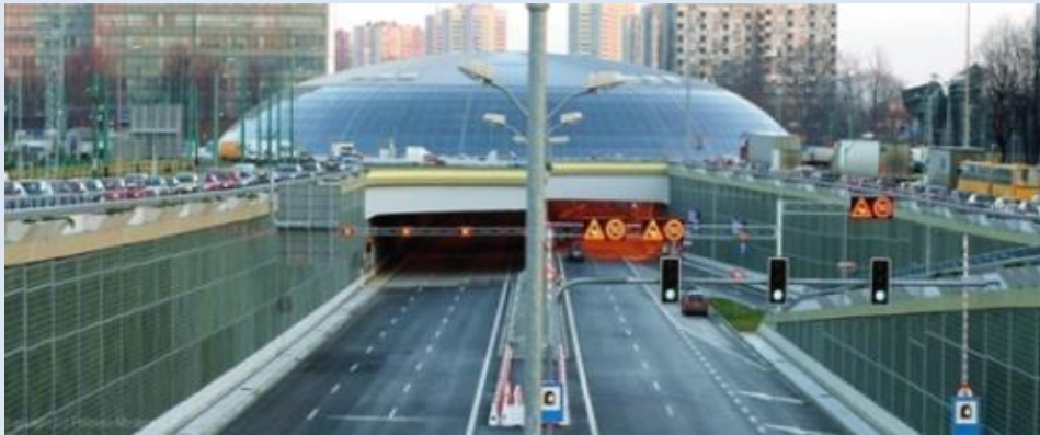
Steel structure cupola over traffic circle in Katowice, Poland 240 tons of steel structure
