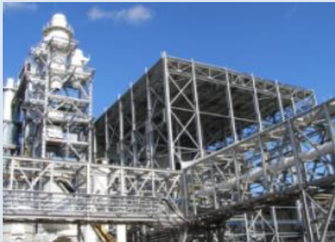
HDF/MDF manufacturing Plant, Poland, 1 750 tons of steel structure
