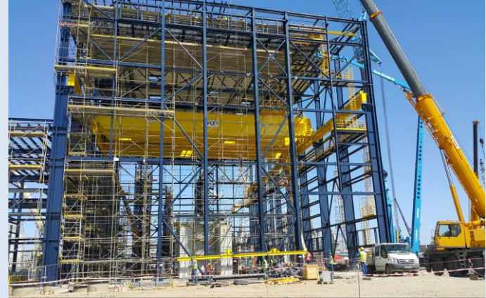
PKN ORLEN Refinery, Poland 3 500 tons of steel structure
