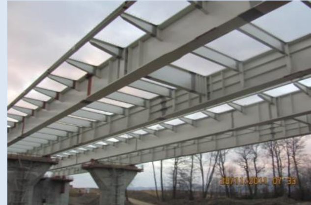
Flyovers ES09 on the way S69, Żywiec - Bielsko Biała, 9 665 tons of steel structure
