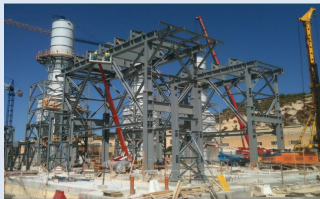
Support structure of the boiler Allborg, Malta 759 tons of steel structure
