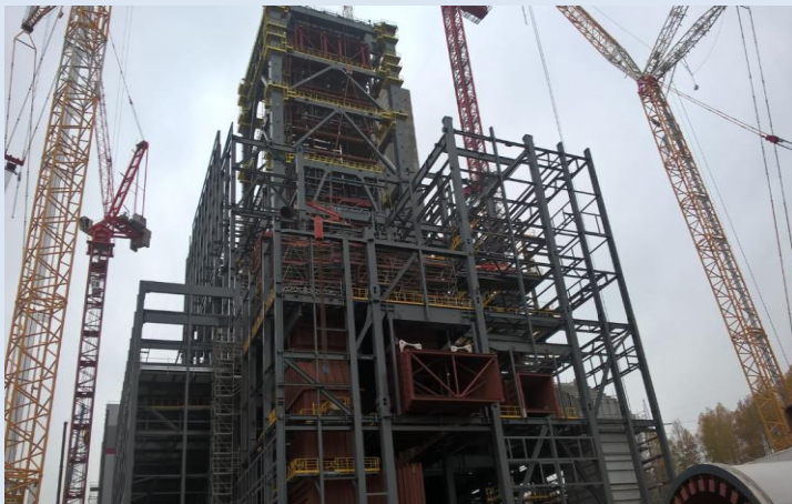
Turów Power Plant, Poland 7 000 tons of steel structure
