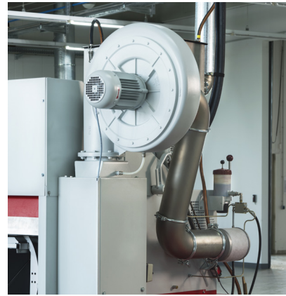
Enhanced drying unit
