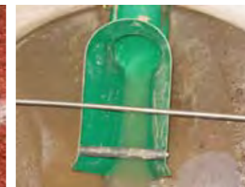
人孔 available from DN 100 (Q max 5,7 l/s) to DN 300 (Q max 94,4 l/s).
