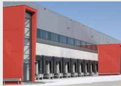
Immogate logistics centre, Munich
