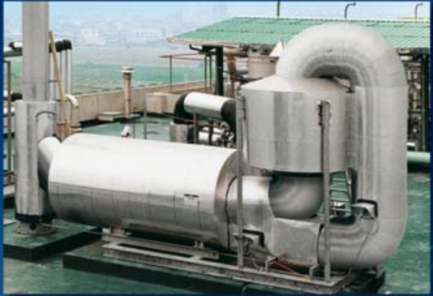
Sizes designed to handle flow rates up to 9 000 m 3 N /h are delivered pre-assembled on a base frame (see sectional diagram); larger units are assembled on site.
