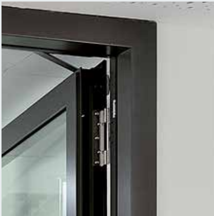
Frame prepared for overhead door closer
