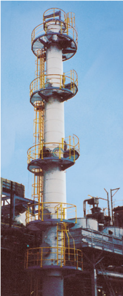
Steam stripper with integral rectification section.
