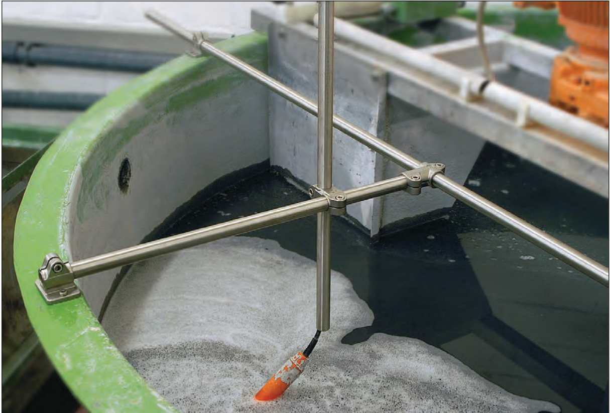
Simple probe fixation in an aggressive environment.
