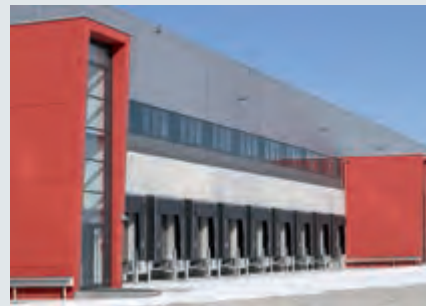
Immogate Logistikcenter, München
