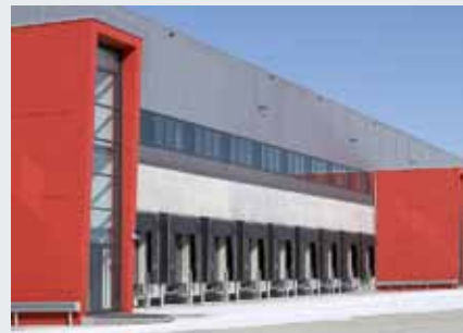
Immogate Logistikcenter, Munich
