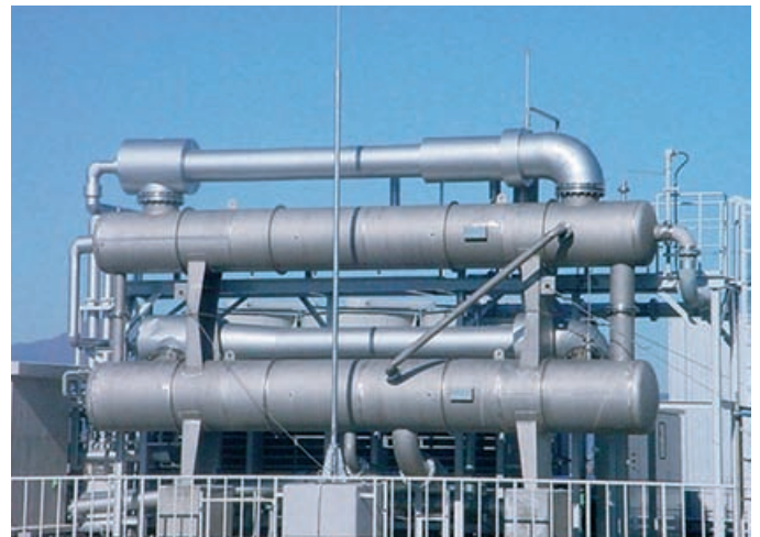
Fig. 5: 2-stage steam jet cooling plant of compact design, cooling 44 m 3 /hr of water from 30 to 10 °C.
