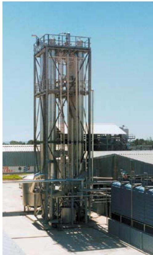
*4-effect falling film evaporation plant for orange juice; evaporation rate: 12,000 kg/h*
