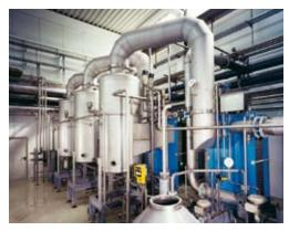
3-effect plate evaporation plant, directly heated; evaporation rate: 3,500 kg/h
