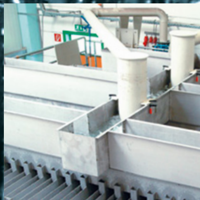
Testing of a through-type distributor
