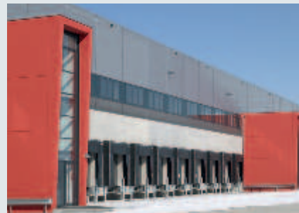
Immogate Logistikcenter, München
