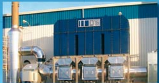
Construction material coating: A 26 000 m 3 N /h RTO with hot water heat exchanger for cleaning the exhaust air from bitumen coating of construction materials.
