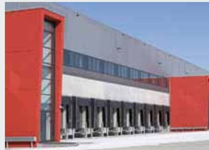
Immogate Logistikcenter, München
