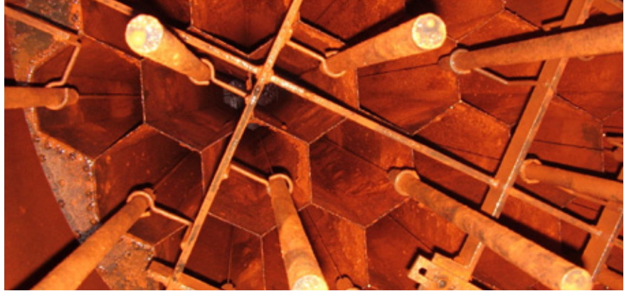
Honeycombs of a wet electrostatic filter
