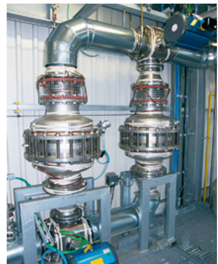
Detonation safety barriers for waste gases according to zone 1
