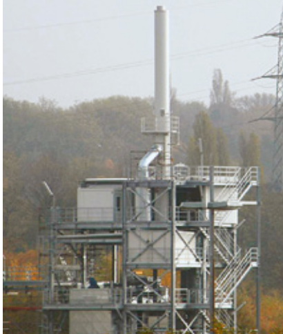
Incineration plant for waste gases containing silane
