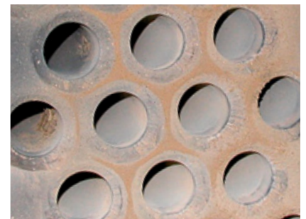
Gas tube boiler for waste heat recovery
