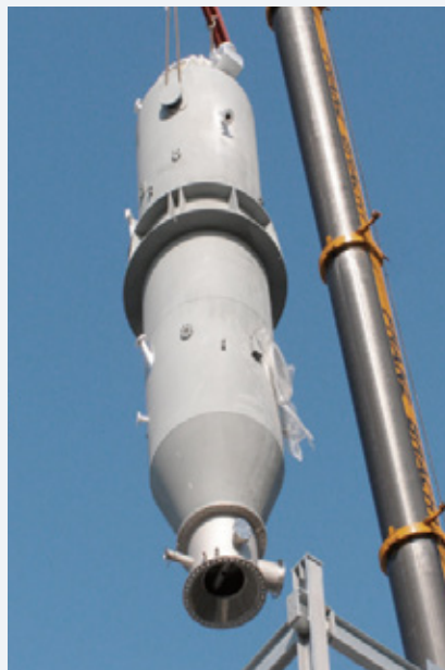
Assembly of a complete, pre-lined combustion chamber with attached, flanged air/water quenching head
