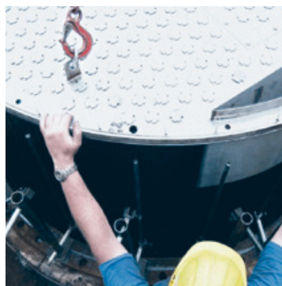
Installation of trays
