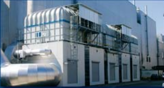
Odour elimination from a foundry: 5-canister RTO version purifying 200 000 m 3 N /h of exhaust air from a Bavarian car manufacturer's light-metal foundry.
