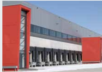
Centro logistico Immogate, Monaco
