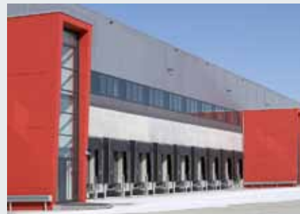
Immogate Logistikcenter, München
