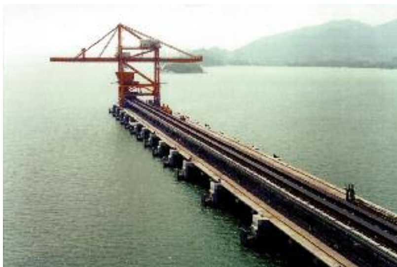
igus® fibre optic cables with 441 m travel. E-Chain®: System E4/4
