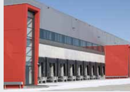
Immogate Logistikcenter, Münih
