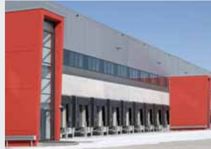
Immogate Logistikcenter, Münih
